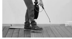
APPLY SANSIN SDF EVENLY BY BRUSH OR SPRAY APPLICATION
